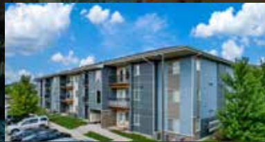
Broadway Apartments Des Moines, IA | Acquired Feb 2024
