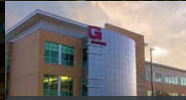
Single Tenant Industrial Office N. Little Rock, AR | Acquired June 2021
